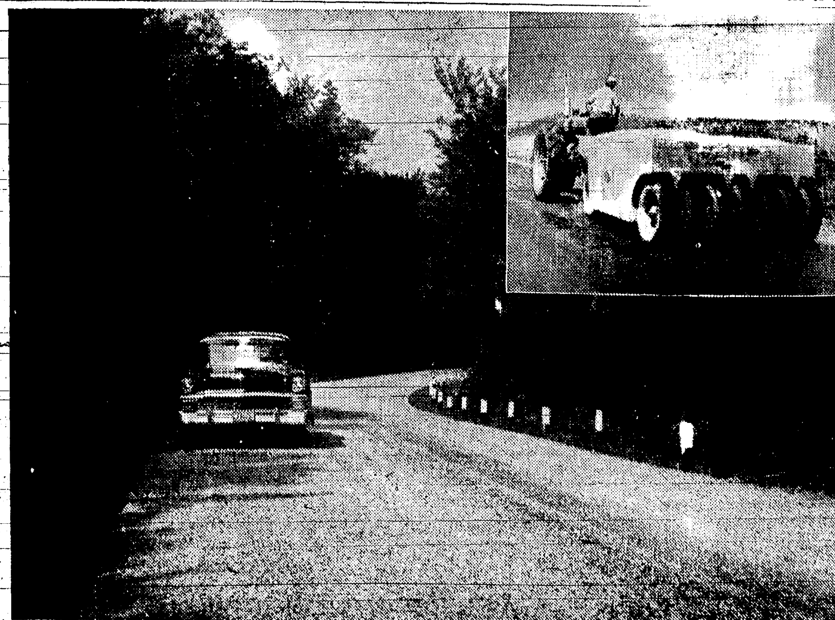
Local traffic can use soil-cement the same day it's laid. No costly delays.
